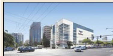
An artist's rendering of the Lock Up self-storage building planned for the current McCully strip mall.
